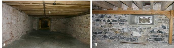
Figure 5. Masonry walls and timber slab system in Beylerbeyi Palace
