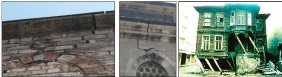
Figure 1. Earthquake damage for masonry and timber structures (Prohitech 2004)
