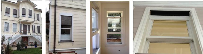
Fig. 1. (a) General view of the Case a house; (b) View of the window system with the aluminium roller shutters are half closed from outside, Case a; (c) View of the window system from inside, Case a; (d) view of the aluminium roller shutter box with the lid of it open, Case a.
