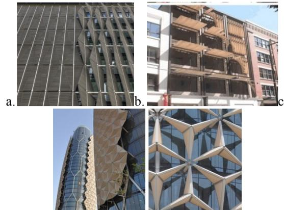
Figure 6: Computerized panels : a. Kinetic façade b. ThyssenKrupp Quarter Essen Building (Germany, 2010) façade, [23-25], c. Al Bahar Tower, overall view from the north and folded panel view
