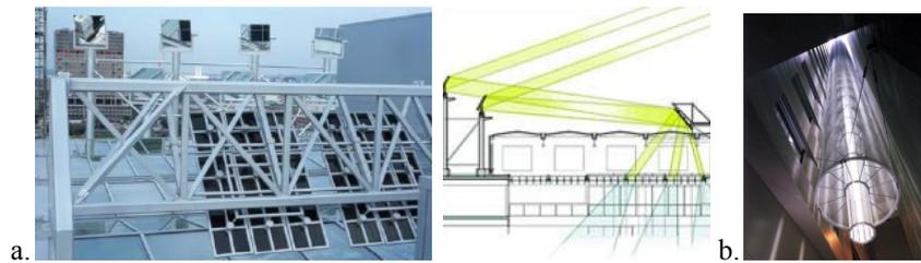
Figure 7: a. Roof mounted mirrors (heliostats) directing sunlight into the building through a skylight, b. A 14-storey height sun pipe [26, Mayhoub 2014]
