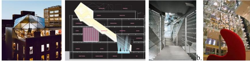
Figure 8: a. Tertiary reflective mirrors (Diane von Furstenberg (DVF) Studio-USA, 2007), b. Milled acrylic prisms in Genzyme Center (USA, 2003) [27, 28]
