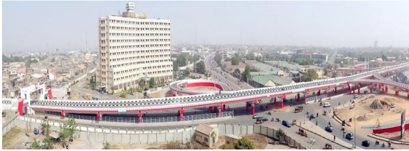
Figure 6. Picture showing the new flyer over bridge at Kofar Nassarawa. (Source: authors field work)
