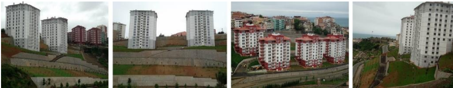
Figure 7. Zağnos Valley and TOKI housing after urban transformation
