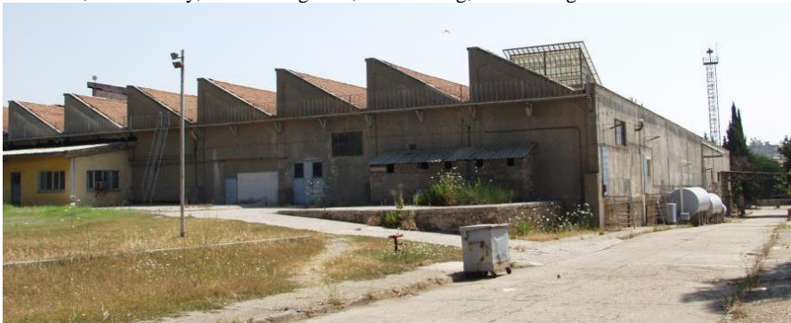
Figure 2. Main Factory Building, exterior view. ( http://kepezdokuma.com )
