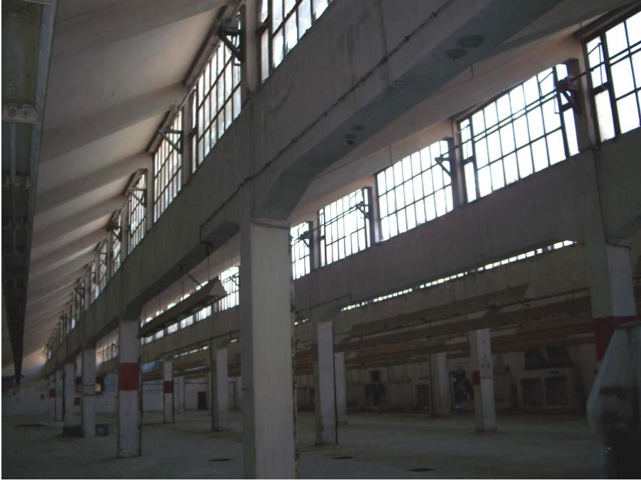
Figure 3. Main Factory Building, interior space. ( http://kepezdokuma.com )
