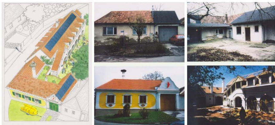
Figure 1. From left clockwise, NAT sketch (areal view), facade (before renovation), courtyard (before renovation), courtyard (after renovation), facade (after renovation); pictures: Löttsch, Deubner
