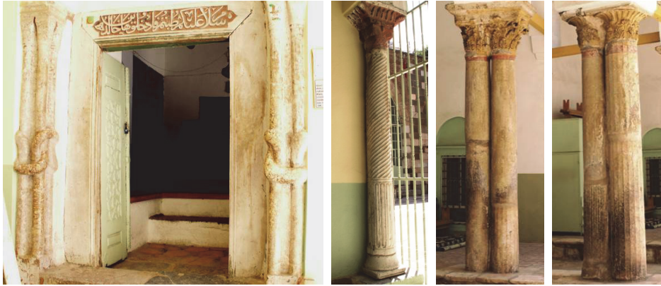
Figure 14. Bilateral Twisted Columns at Entrance of Tomb (Left) and Reused Columns-Columns Heads (Right)
