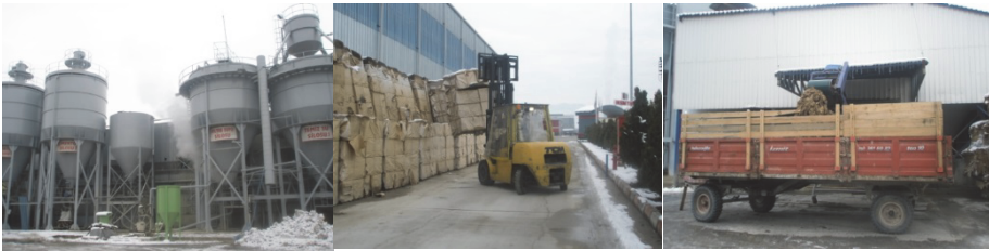
Figure 1.Cement and Water Silos (Author 1 , H. Bozkurt Archive, 2013)
