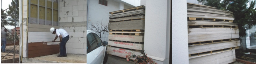
Figure 17. Fibrecement Board Construction (Hekimboard Application Movie, 2013)
