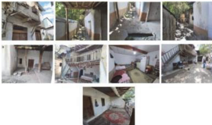
Figure 7. The number 10 house of Beybağı Neighborhood
