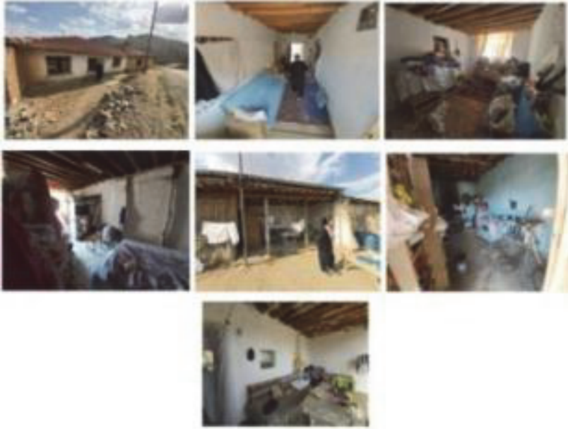
Figure 14. The number 14 house of Beybağı Neighborhood
