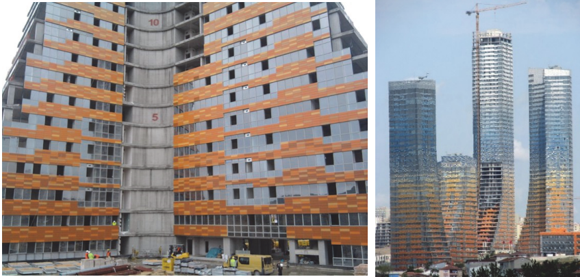
Figure 9 Varyap Meridian Facade Construction ( http://gezginharitaci.blogspot.com/2013/04/varyap-meridian.html ).
