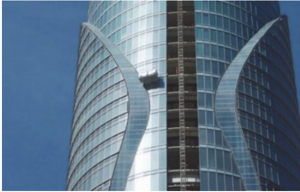
Figure 10 Spine Tower Facade Construction ( http://www.saytekno.com/ ).
