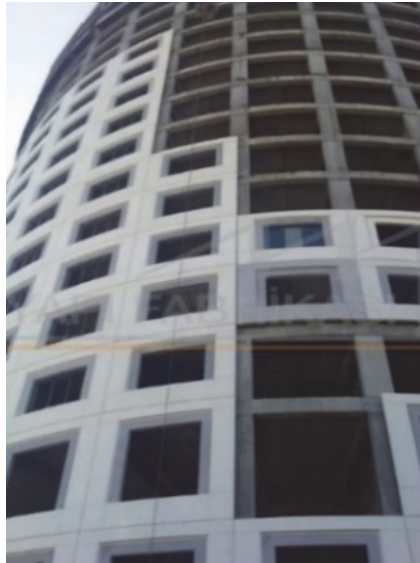
Figure 11 Orya Park Facade Construction ( http://www.yapifabrikasi.com.tr/ ).
