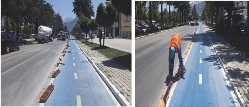
Figure 1. Dismantling of Bicycle Lanes (Hürriyet, 2018).
