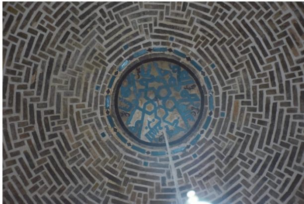
Figure 2: The dome braiding at Tahir and Zuhre Mosque and the tile panel at the center of the dome
