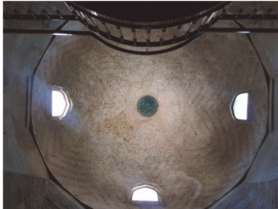
Figure 4: The dome of the Beyhekim Mosque
