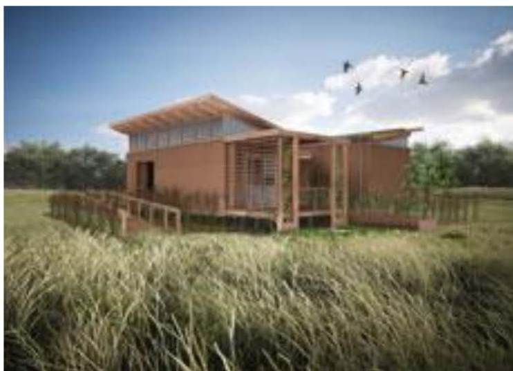
Figure 5. Computer-generated rendering of the Team Maryland house, an example of a low-pitch roof with PV panels. This house won first prize in the 2011 Solar Decathlon. (Courtesy of the University of Maryland Solar Decathlon team)
