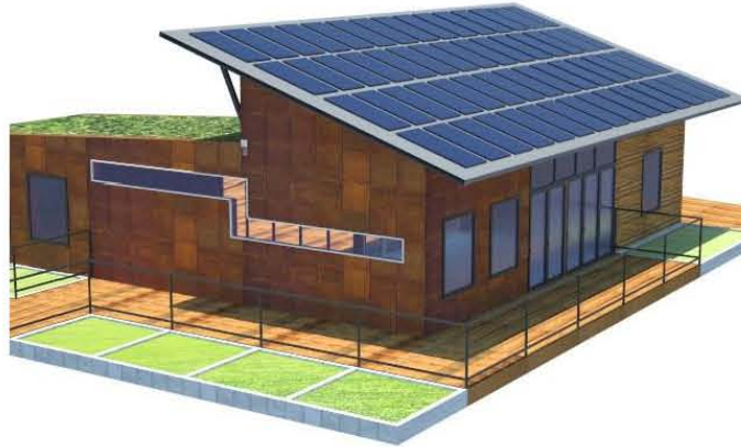
Figure 6. An early version of the Team Kentuckiana house, showing the integration of the PV array on the south-facing roof
