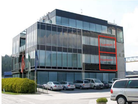
Figure 8. FIBAG - Office building with two test rooms (marked)
