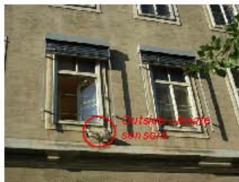
Figure 6. VUT – Façade with climate sensors
