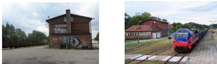
Figure 11. 12. Kartuzy - Station buildings
