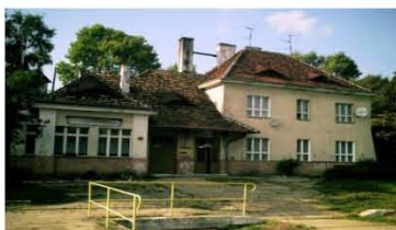
Figure 13. Babi Dół station building
