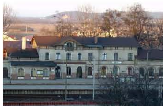
Figure 8. Reda station building
