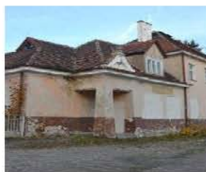
Figure 18. Wieżyca railway station building
