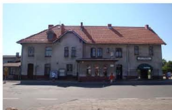
Figure 7. Puck station building
