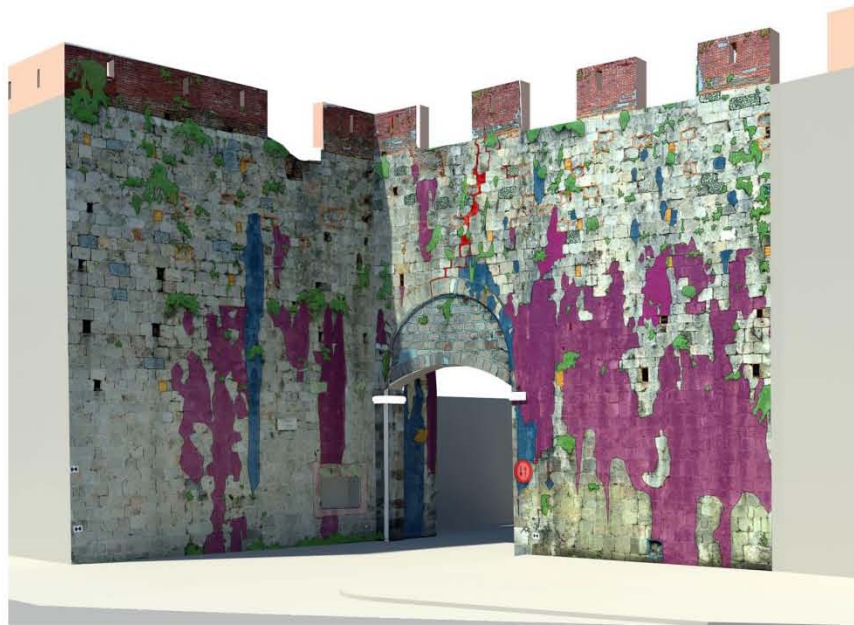
Figure 7. Pisa (Italy), walls of the city – 3D model texturized with the deterioration mapping
