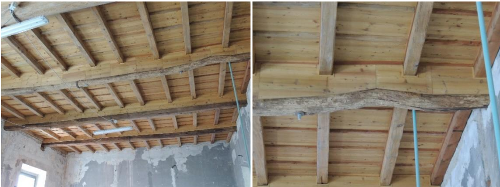
Figure 4. The insertion of new horizontal structures on old timber beams, Ex caserca Calchi, Pavia, Italy. The historical beams are reinforced by the addition of new beams (photo: Andrea L'Erario, 2014)
