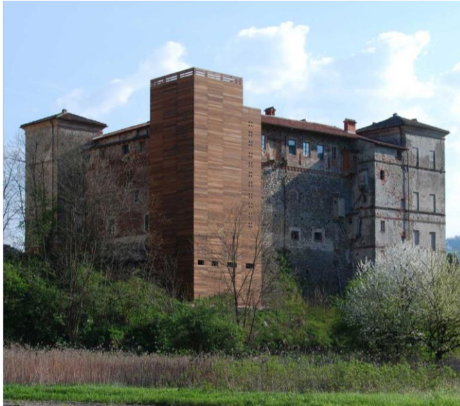
Figure 5. Saliceto Castle, Italy. Restoration project by Armellino&Poggio Architetti Associati, 2011. The new tower, made with a steel and timber cladding self-supporting structure, is well noticeable from the historic castle.
