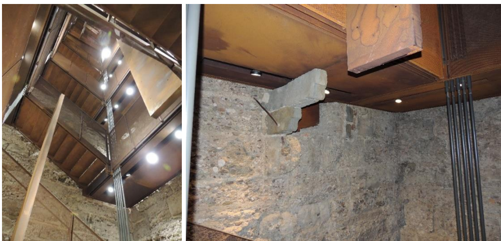
Figure 2. The new stairs inside Bernabò Visconti Tower (Castle of Trezzo sull'Adda, Italy, project: Lorenzo Jurina and collaborators) is a good example of reversibility and integration between old and new structures (photo: Andrea L'Erario, 2014)
